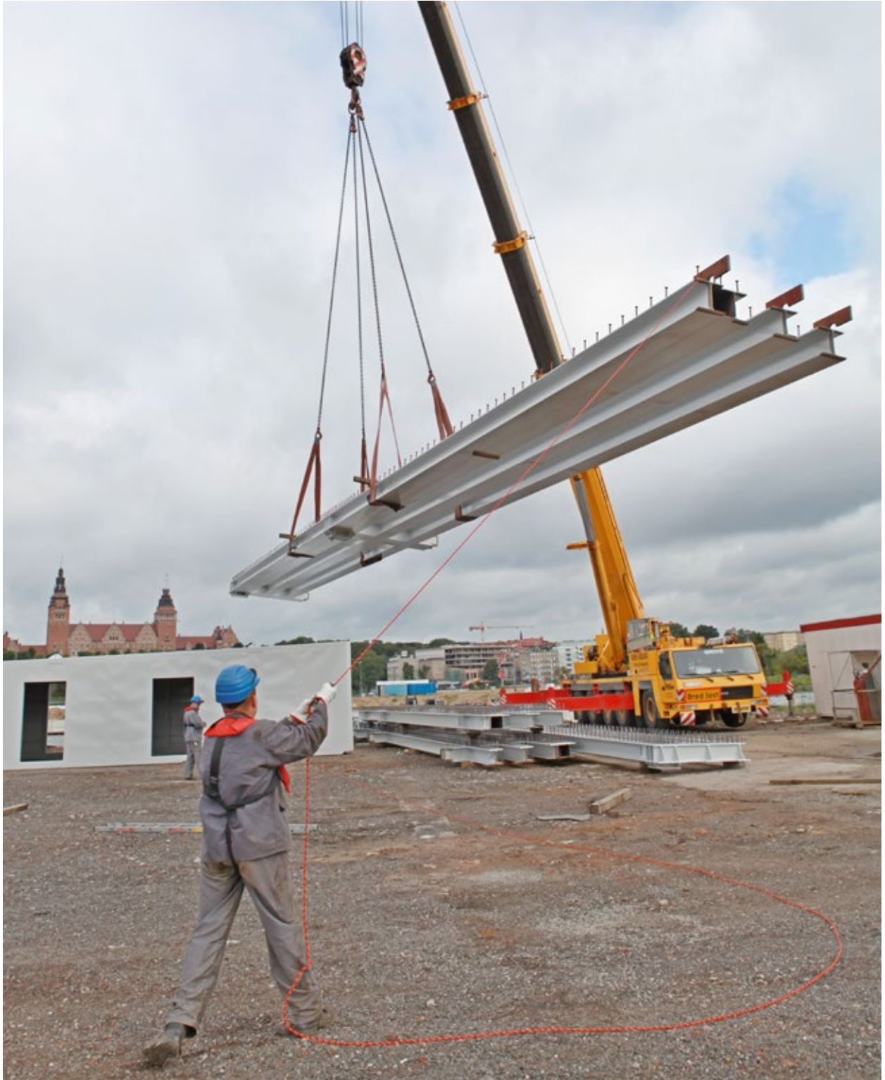
Steel bridge construction
