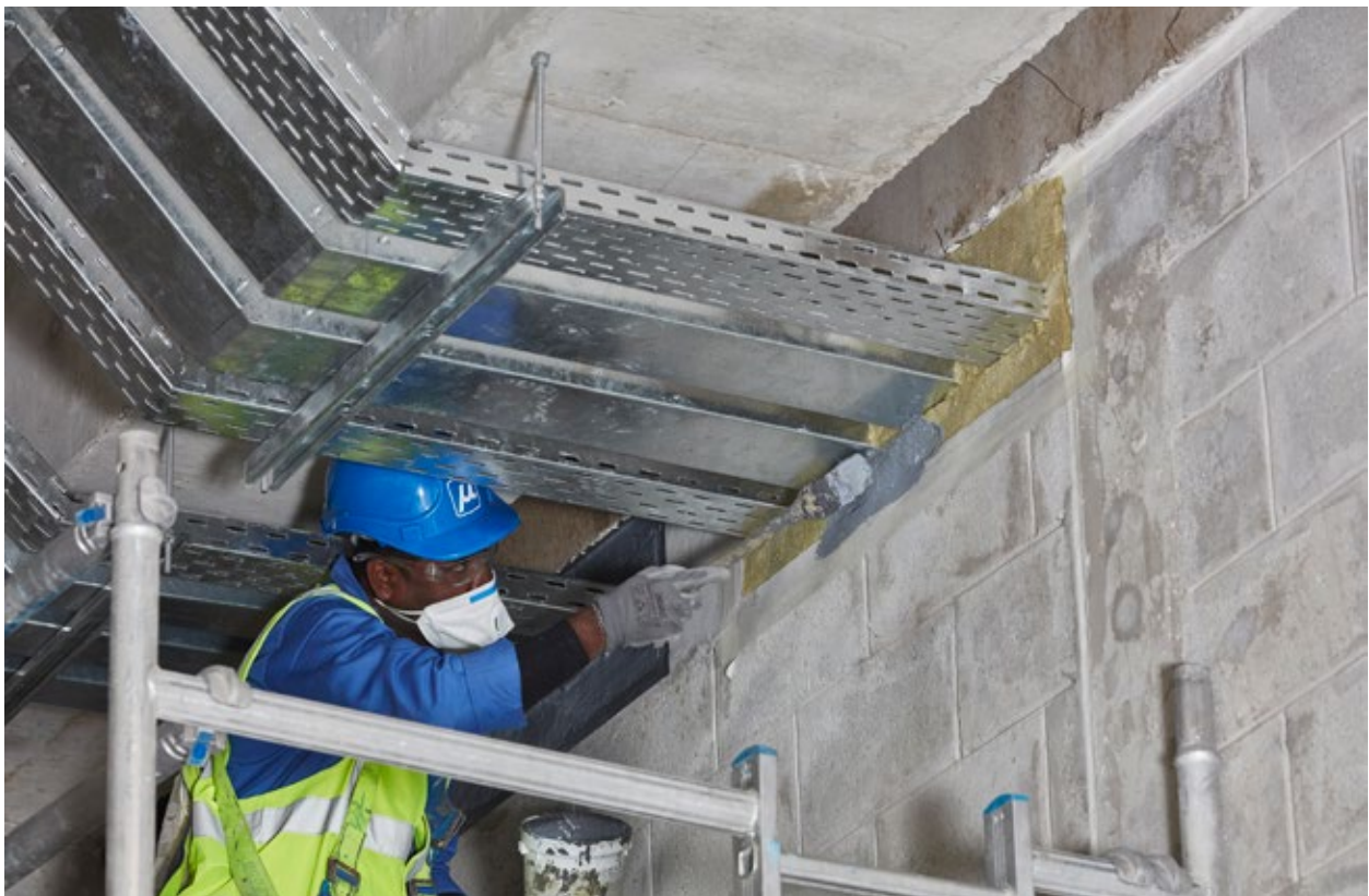
Applying passive fire protection
