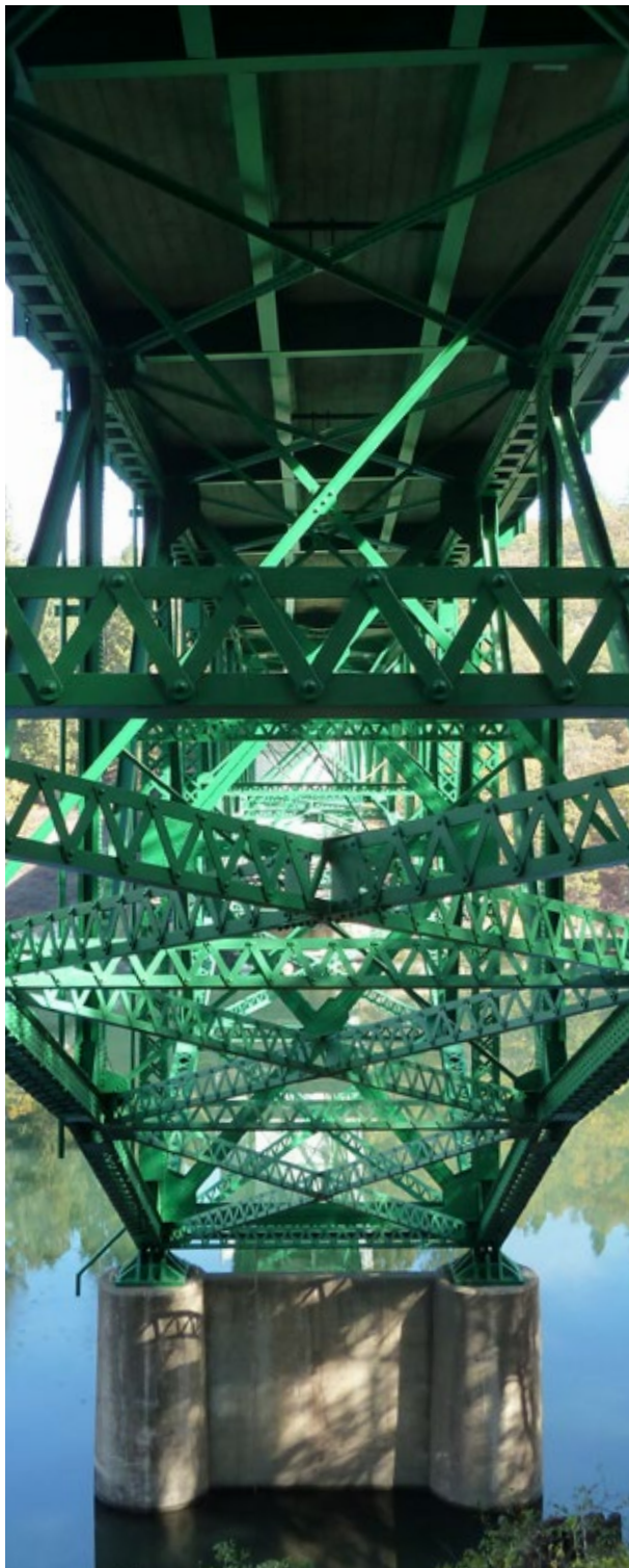
Coating of the Lake Britton Bridge, California/USA
