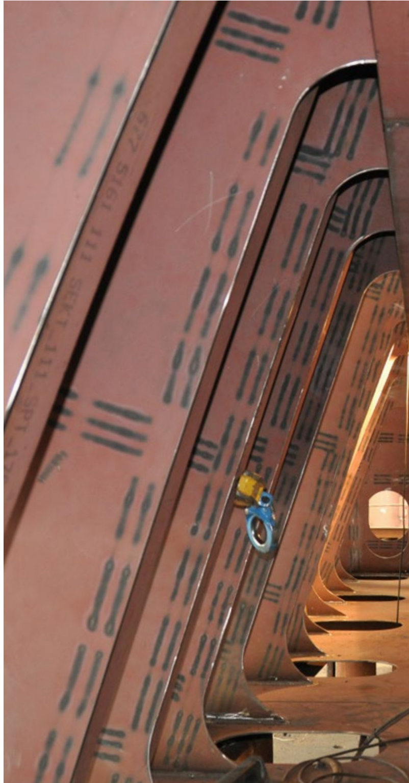
Steel construction in Gdansk, Poland
