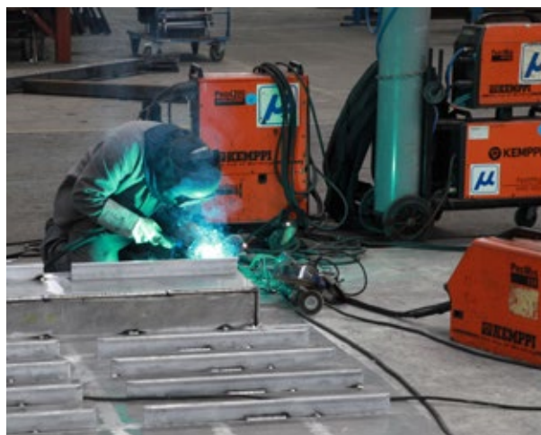
Steel construction work
