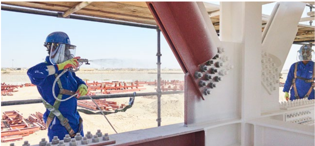
Applying passive fire protection
