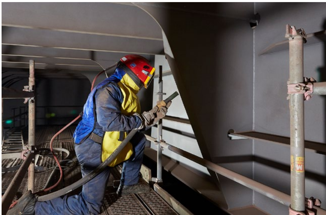
Steel construction work
